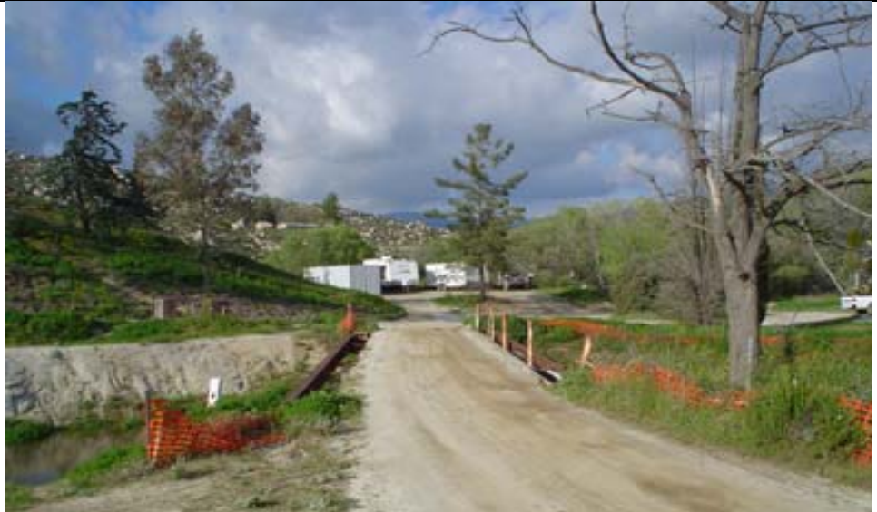
The Road into "Base Camp" at MotoVentures
